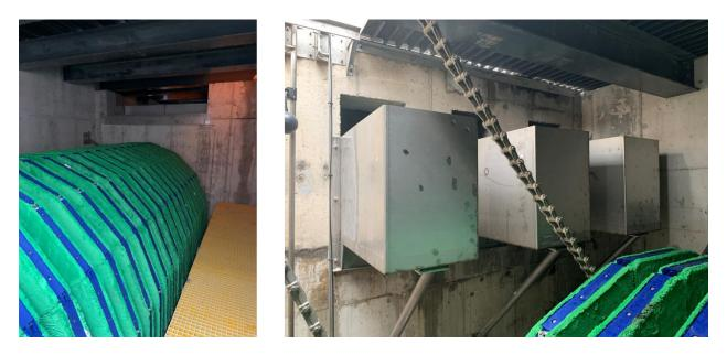
Figure 11: Inside view of the AquaPrime Filter unit showing influent weir
